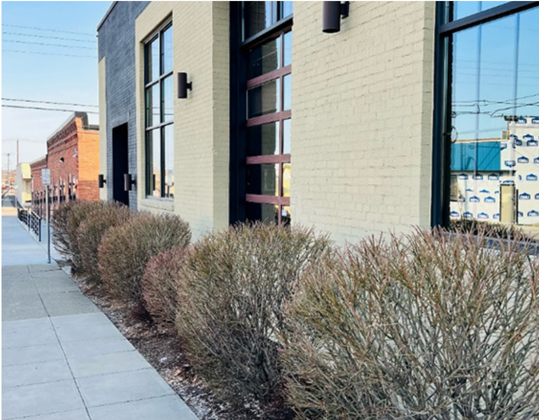
Spokane Art School's new UD location at the northeast corner of Sherman and 2nd Avenue.
