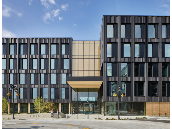
Left: Aerial view from Gonzaga University (foreground) of the Spokane River, downtown Spokane (at right), and the University District and hospital district (at left) Above: The zero-carbon, zero-energy Catalyst Building, part of the South Landing EcoDistrict
