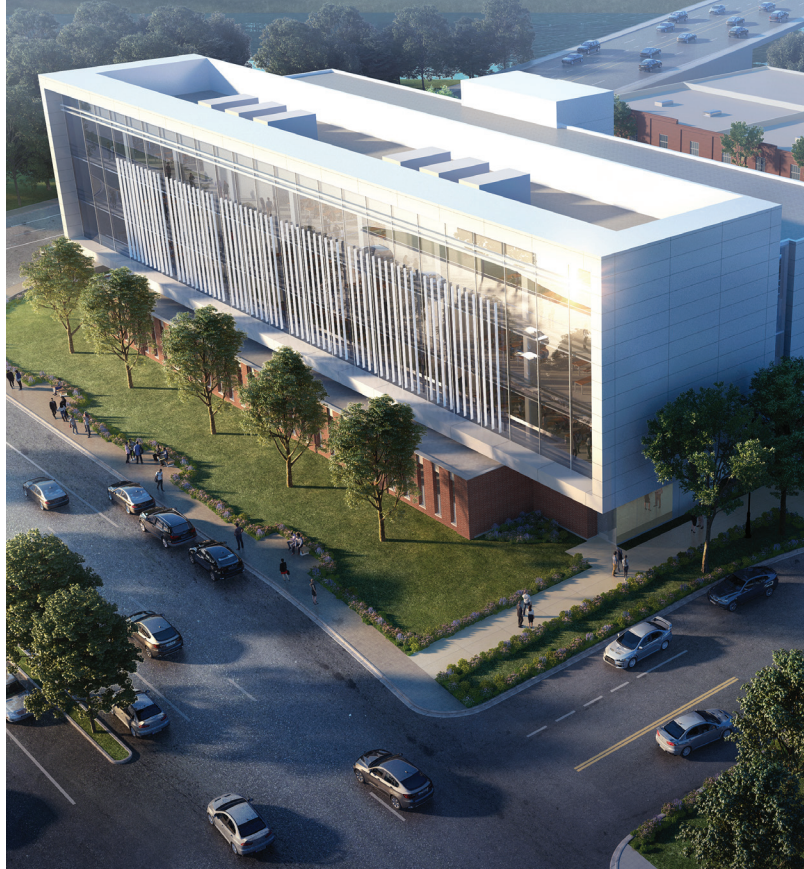
Above: The University of Washington School of Medicine-Gonzaga University Health Partnership's 80,000-square-foot building on the new "Health Peninsula" is set for 2022 completion
