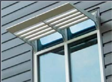
McKinstry engineers performed more than 40,000 energy model simulations during building design.
