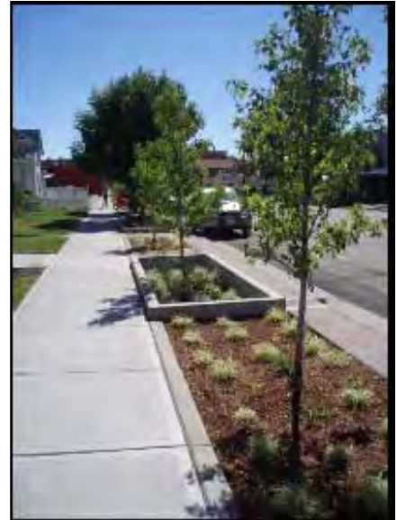
Figure 11: Finished storm gardens, Broadway Ave
