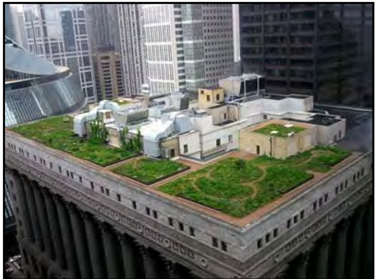
Figure 6: Green Roof, Chicago, IL
