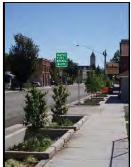
Figure 12: Finished storm gardens, Broadway Ave
