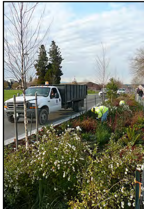
Figure 19: Street side bioswales, High Point Neighborhood Seattle, WA
