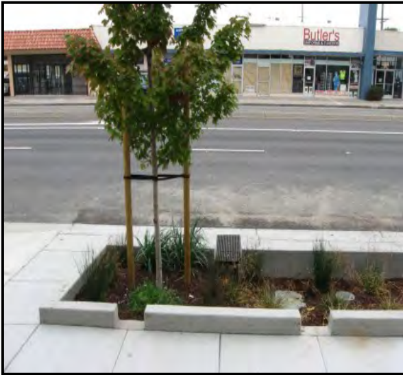
Figure 3: El Cerrito Storm Garden
