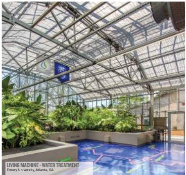
LIVING MACHINE - WATER TREATMENT Emory University, Atlanta, GA
