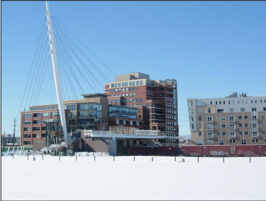
Figure 14: The Millennium Bridge, Denver, Colorado
