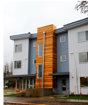
3-story Apartment surface, tuck-under parking
