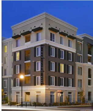
5-story Wrap interior structured parking
