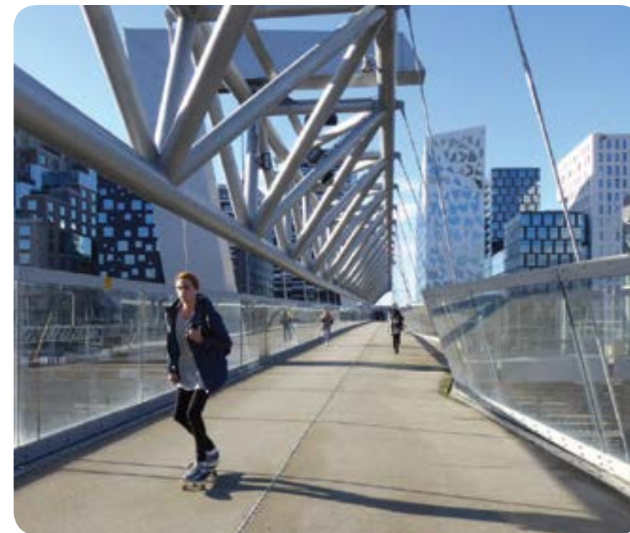
—The pedestrian bridge in Bjørvika, Oslo Norway.
