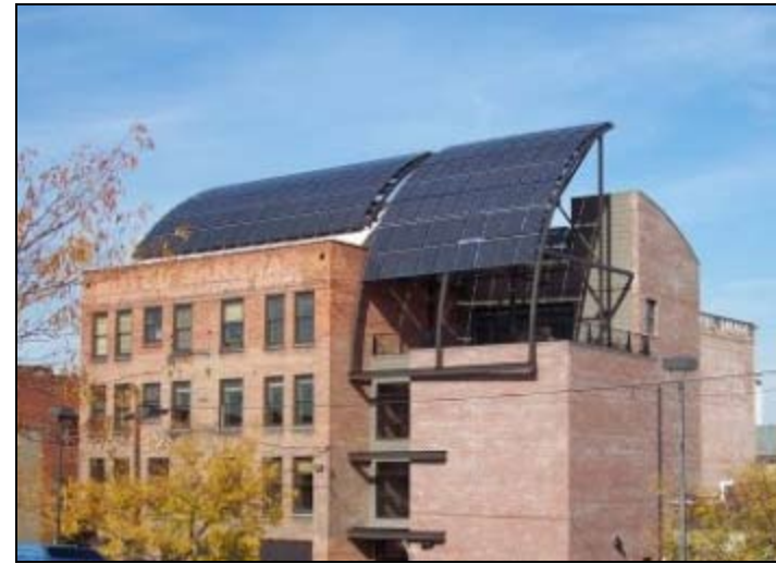
Saranac Building: Solar Panels • Source: http://www.solaripedia.com
