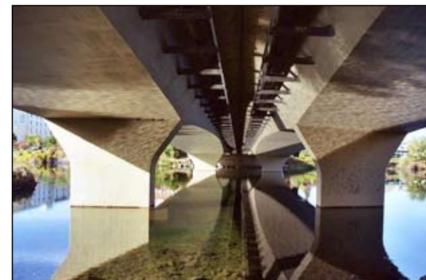
Division Street Bridge • Source: flickr.com/photos/80651083@N00/104439912/in/photostream/
