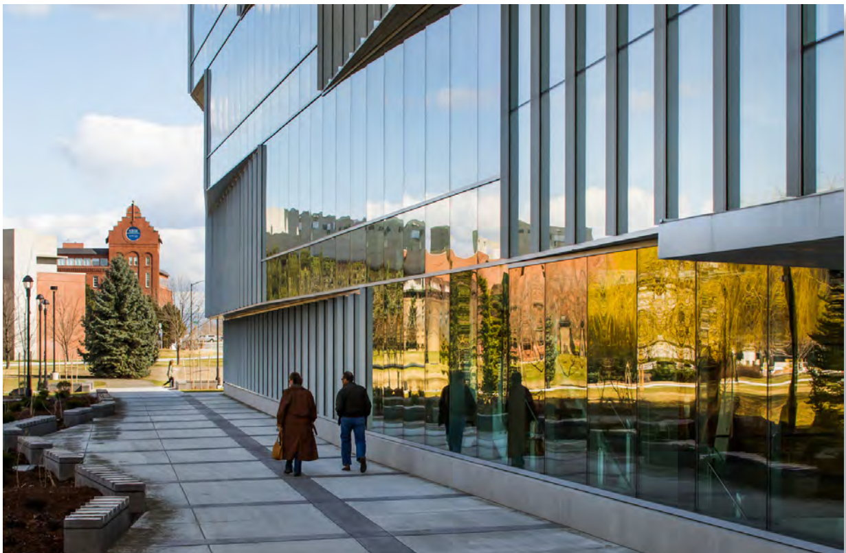
Figure 3.3 Campus Reflection, PBS Facade
