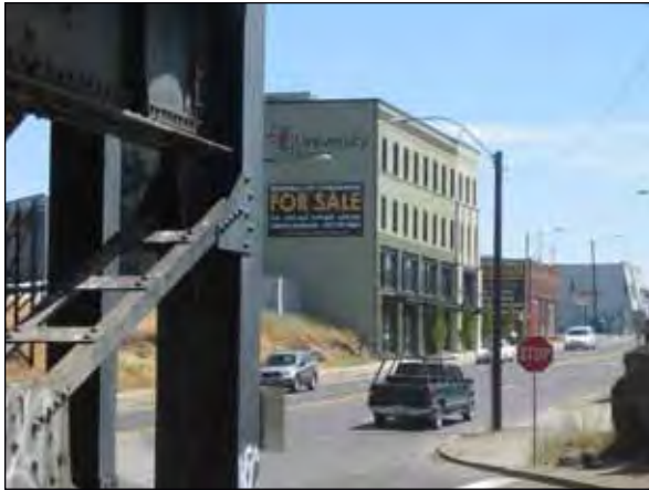
The Edge Lofts on Sprague Avenue are tapping latent demand for housing in Downtown Spokane.
