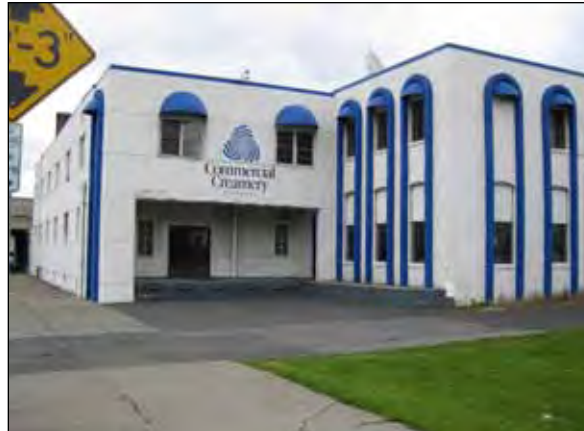
The Commercial Creamery Company is one of many light industrial buildings still in use south of the railroad tracks.
