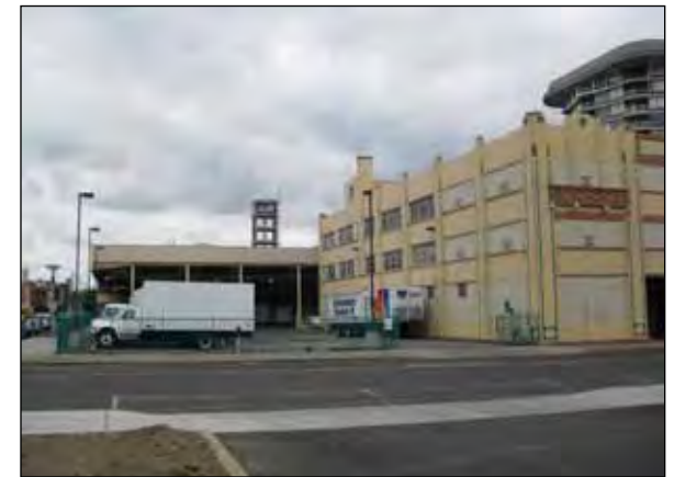
The Old Greyhound Station Site is currently used for staging and storage by the Spokesman-Review.
