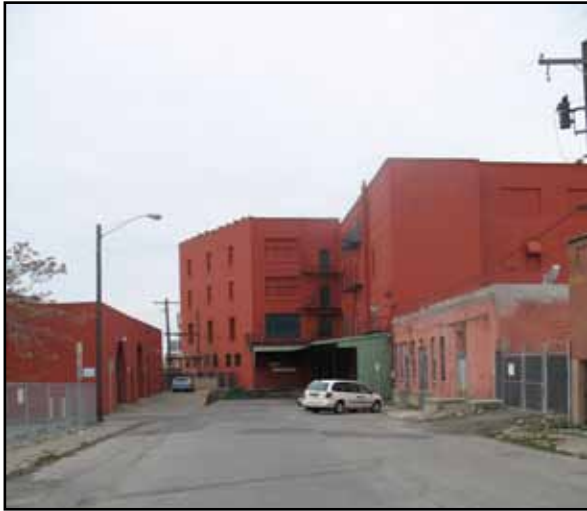
A-Economy Building is a mini-storage warehouse operating in the South University District
