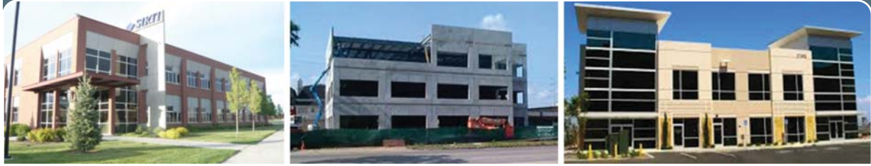
Innovate Washington SIRTl Concrete Tilt-Up Office: Under Construction Concrete Tilt-Up Office: Completed
