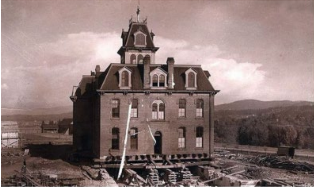
Caption: Gonzaga's College Hall under construction. Image courtesy SpokaneTalk.
