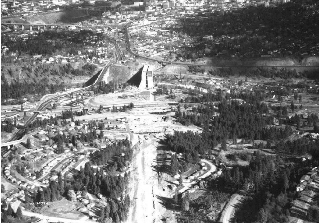
Caption: The construction of I-90 through Spokane. Image courtesy of the Northwest Museum of Arts & Culture.
