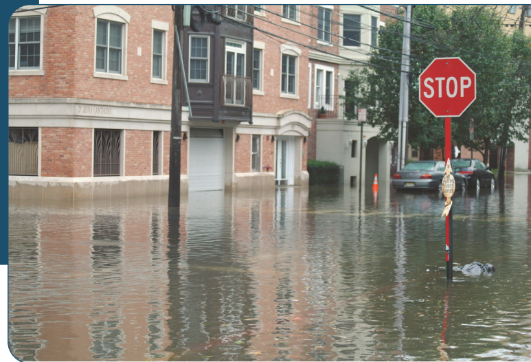
Flooded street in Hoboken following Hurricane Sandy (2012)
