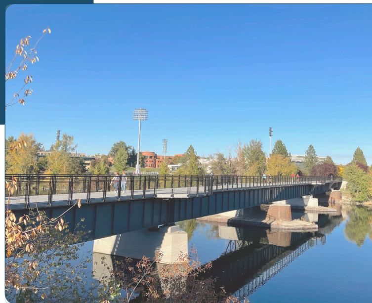
Renovated Don Kardong Bridge
