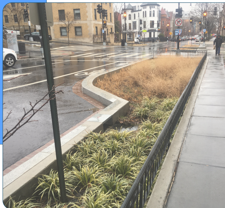
A bioswale in Washington, DC
