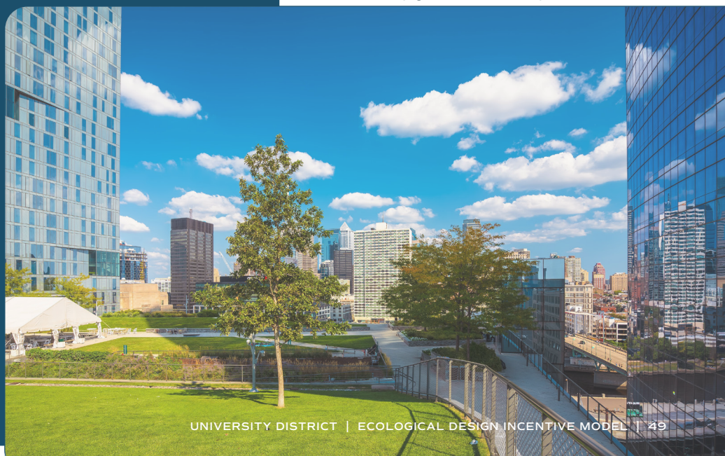
CIRA Park rooftop garden in Philadelphia
