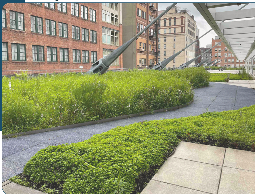
Green rooftop at the David L Lawrence Convention Center in Pittsburgh, PA
