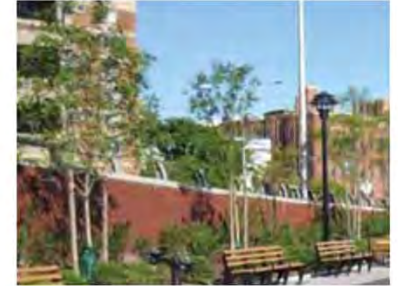
The design for Harlem River Greenway replaced collapsing steel sheeting with porous edges (including gabion baskets filled with oyster shells) to help clean the river water, restore floodplain functions, improve near-shore habitat and allow a safer approach to Manhattan by kayak.
